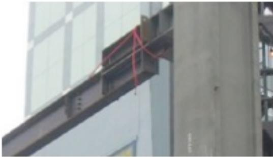
Figure 4: ‘Dog-leg’ beam connection
